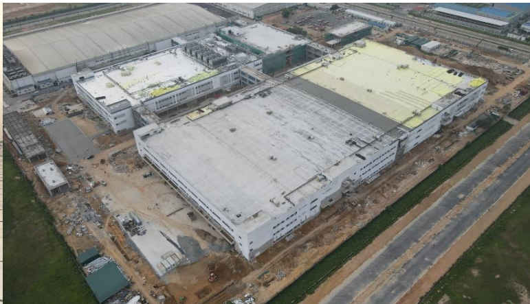
Compal Factory (Ba Thien I Industrial Park, Vinh Phuc)
